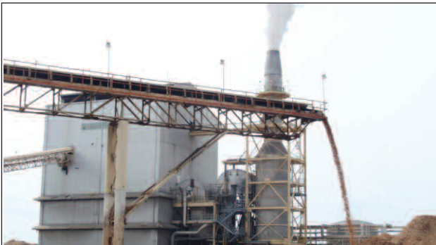
From the transfer tower, the chips are conveyed to a pile for storage. They are further screened and washed before being sent to the pulpmill. Refuse wood (bark and sawdust) is burned in the boiler and the steam is used to cook chips and dry paper.
